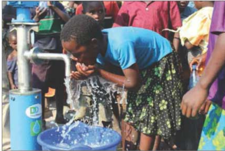
A young girl drinks water from a newly installed LifePump in Malawi, Africa. Photo provided by Design Outreach.
